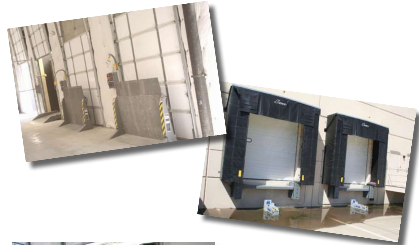
◀ Lower – A release of the lever on the LoadHog dock bridge enables it to softly lower in place to the truck trailer bed, enabling shipment of positioning arms at the Stryker manufacturing plant.
